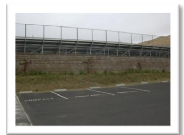
Retevment Wall and Bleachers
