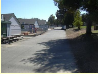
Hamilton Fire Lane
