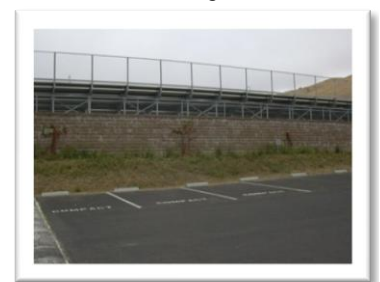
Retentment Wall and Bleachers
